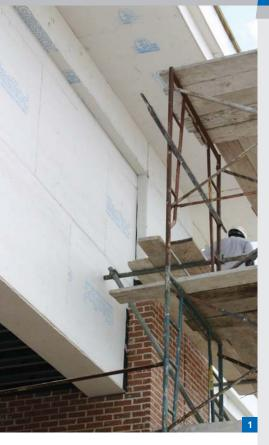
BPB's patented Enhanced Glass Reinforced Gypsum Technology, developed almost 20 years ago, yields a high performance, sustainable exterior gypsum sheathing that provides superior mold and mildew resistance in tropical climates and up to 6-months protection from weather exposure. BPB was awarded an additional patent in 2003.
