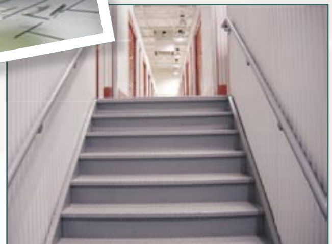
Stairway to second floor. Existing lighting and air conditioning is visible on the ceiling.
