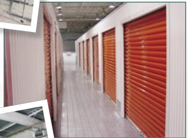
Second floor, showing internal hallway and doors, and warehouse ceiling.
